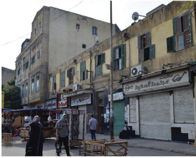
Building NO.1,2 (conditions before intervention)
