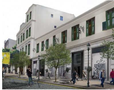
Building NO.1,2 (conditions before intervention)
