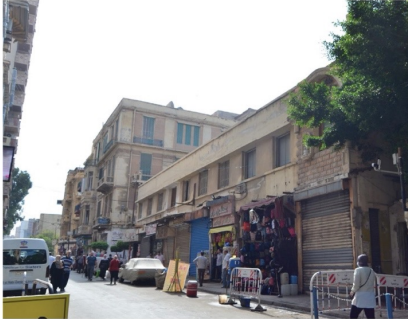
Building NO.6 (conditions before intervention)
